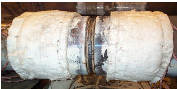
Figure 2. Welding a Cr-Mo steam pipe in a power station [4,9]
